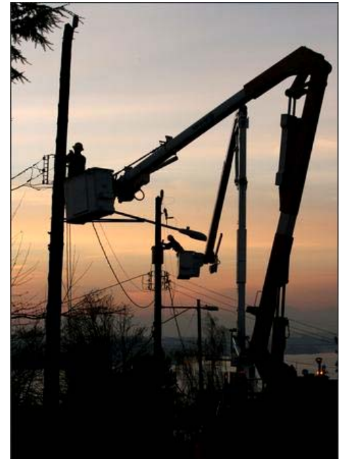
Repairing the damage after 2006 windstorm. Credit: Grant M. Haller/Seattle Post Intelligencer
