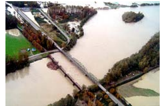
Credit: FOIA to the US Army Corps of Engineers, Seattle District.
