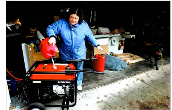
Alverna Palmer puts gasoline in the generator. The Carnation family finally saw the light Sunday night, when crews restored heat and light to the beleaguered community. (December 25, 2006)
